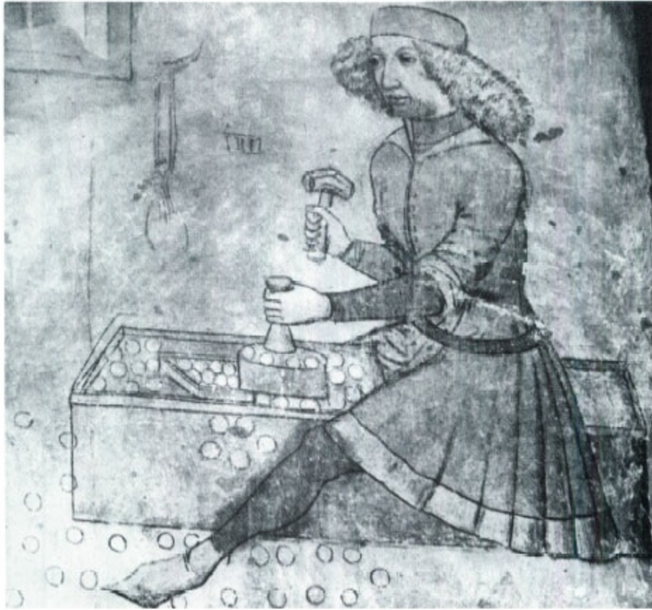
A fifteenth-century Czech coiner at work, striking coins from silver blanks. This was extremely delicate and demanding work, for each coin had to be struck perfectly with one blow.
