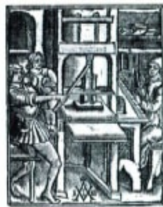
The earliest illustration of a printing press, 1507.
