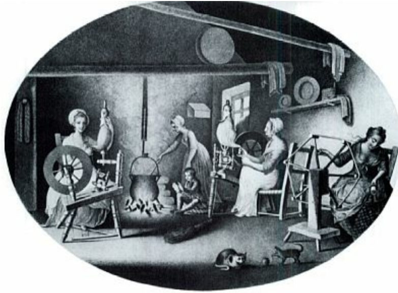
The homespun textile industry. Here, a view of workers preparing flax in Ulster. On the left, spinning the yarn; centre, boiling it; and right, reeling it for use.
